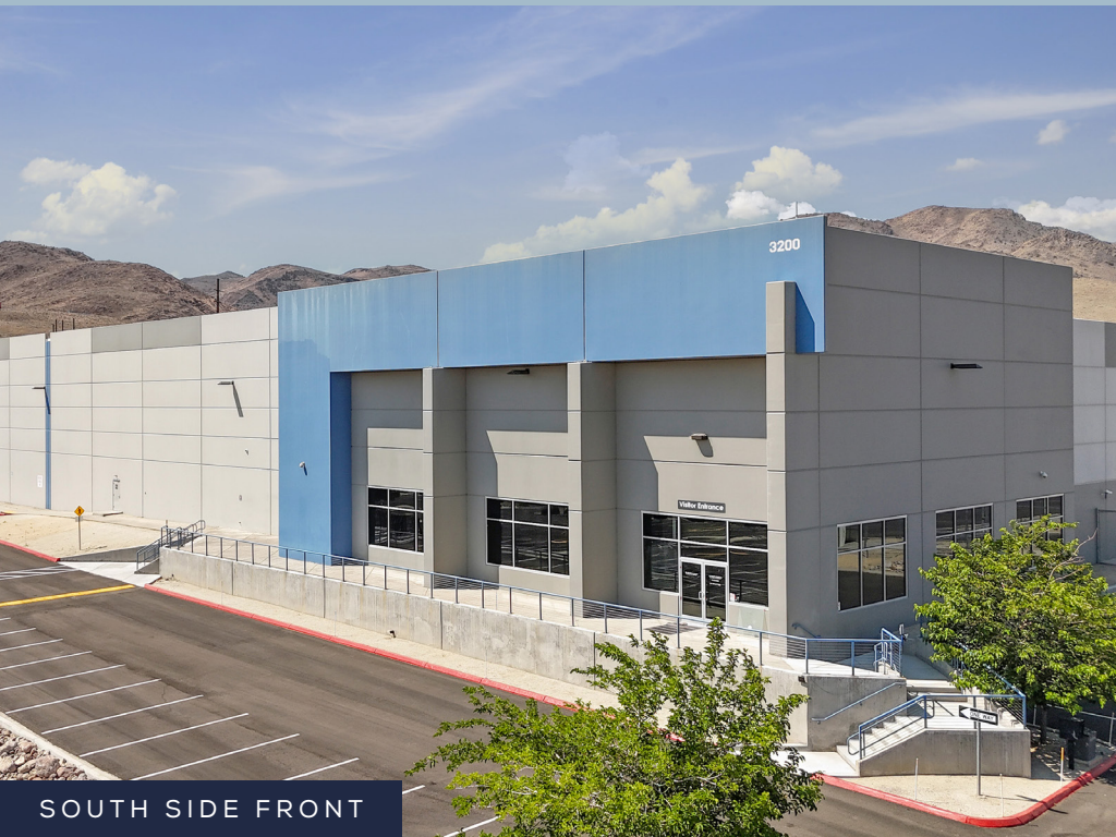
SOUTH SIDE OF BUILDING LOOKING WEST
